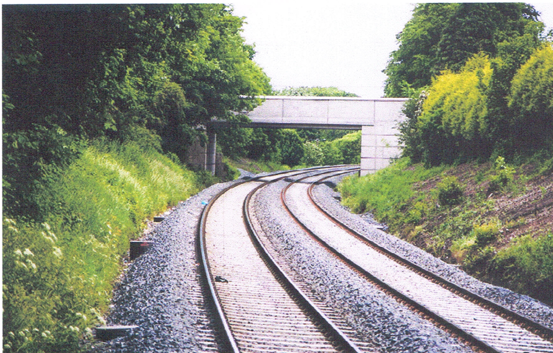
Figure 7.5 Modern re-inforced concrete bridge at Lambeg, NIR.
