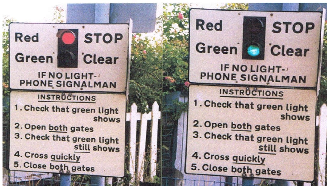
Figure 3.3 Miniature Stop Lights, Westbrook Lane UWG LC near Collingham, Lincs, showing both operating conditions. Note the 'home made' light shield fitted to the right hand side.
