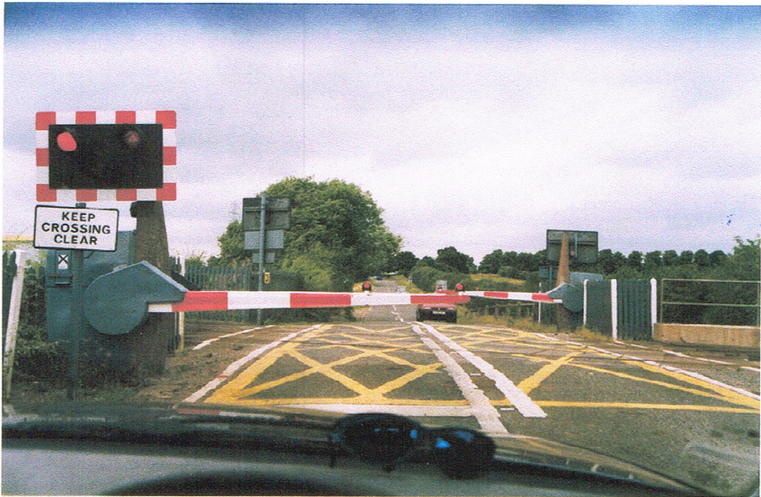
Figure 3.9 Willington, AHB LC on the Derby Uttoxeter line; The waiting period. Seen through the windscreen of the author's car. Note the 'Yellow' box road markings.
