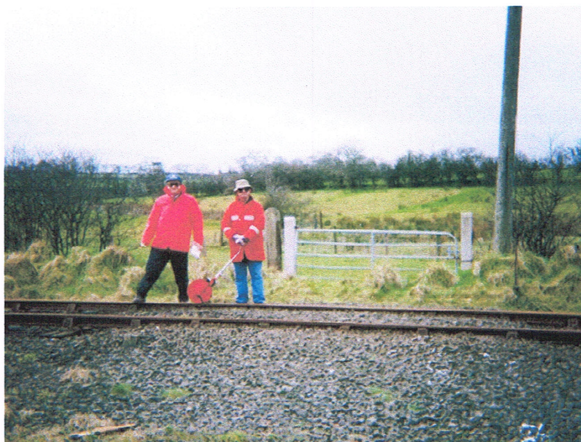
Figure 3.1 Typical Accommodation level crossing, NIR, on the Bleach Green to Antrim line near Doagh; note the lack of any decking for the user.
