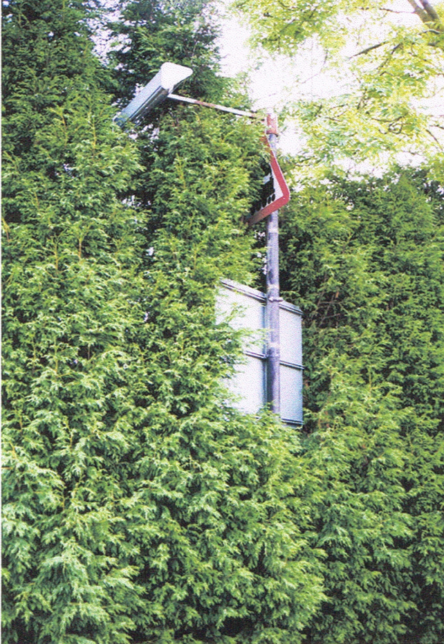
Figure K.13 Bank Foot AOCL LC (top), and Callerton AOCL LC (lh side), TMR; England is a green and pleasant land..... particularly when it comes to obscuring vital road signs with vegetation.
