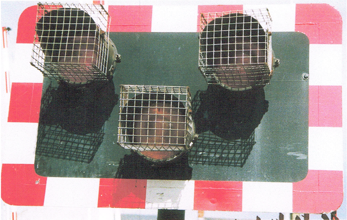
Figure K.19 William Street MCB LC, Lurgan, NIR, County Armagh (top) and Howden AOCL LC, TMR (lh side); Vandals are a problem in a lot of places and are a sad reflection on life in the '90s. In Northern Ireland and particularly in the Lurgan and Portadown areas special measures are needed.
